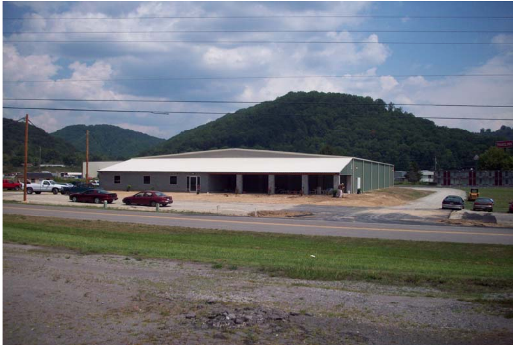
After a season in a temporary facility, the new Appalachian Harvest packinghouse was completed in July, 2008, in Duffield, VA.
