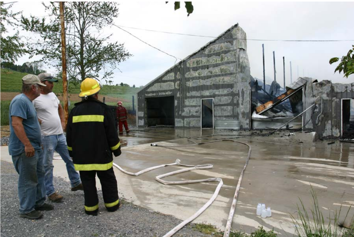
An electrical fire destroyed the packinghouse in May, 2007.
